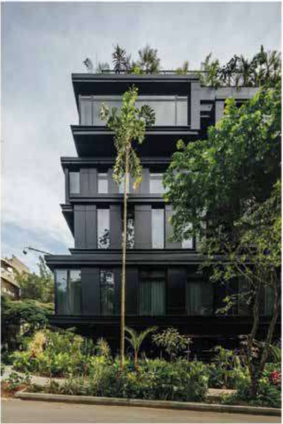
The Click Click hotel, above, and office building Antejardín, opposite, both designed by Plan-B, use cross-ventilation and native plants to reduce internal temperature and energy consumption
